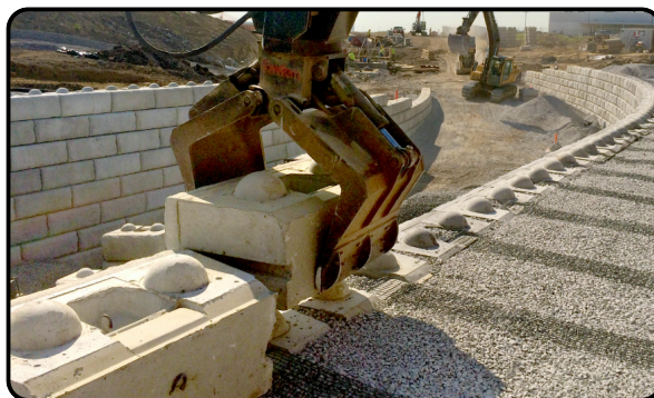
Figure 13 - Infill Stone and Geogrid Layers Shown During Installation
